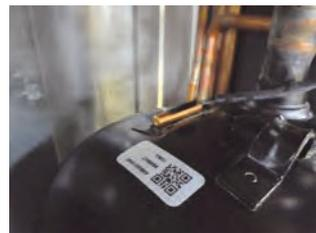
Remove the Thermistor (Comp.temp)
