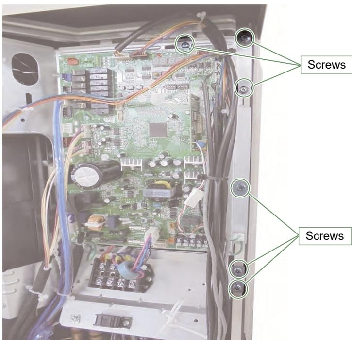
Remove the 6 mounting screws.
