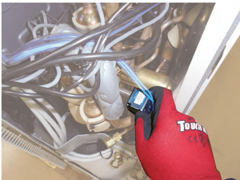
Remove the SOLENOID COIL
