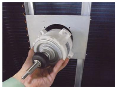
Remove the FAN MOTOR.
