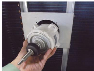
Remove the FAN MOTOR.
