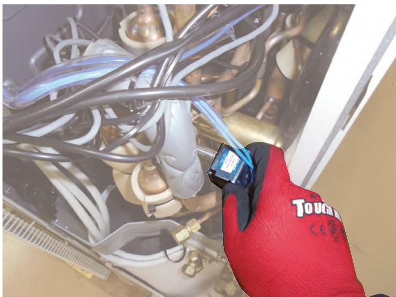
Remove the SOLENOID COIL
