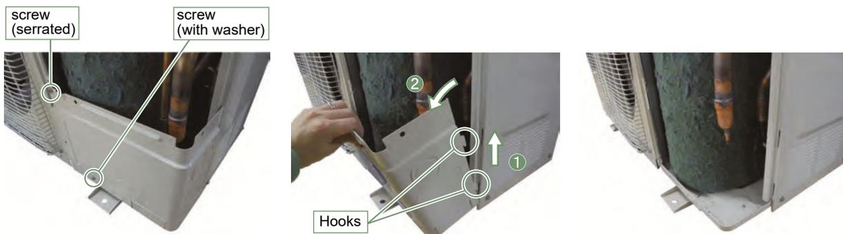
Remove the mounting screws.
