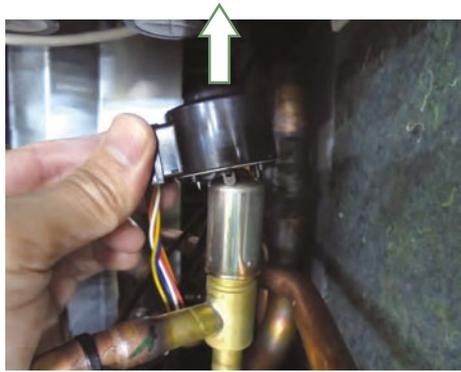
Remove the EEV coil by hand.
