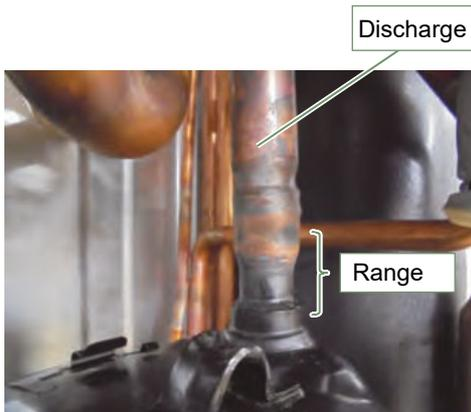
Cut the Discharge pipe in this range.
