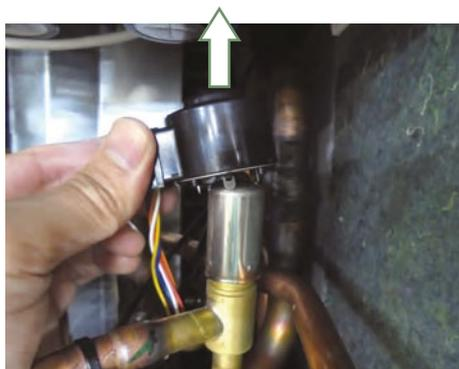
Remove the EEV coil by hand.
