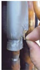
Remove the Thermistor clip and Thermistor(Discharge).
