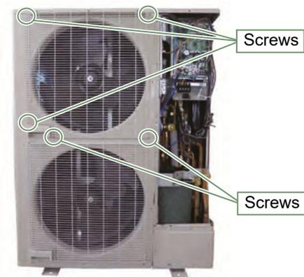
Remove the 5 mounting screws.
